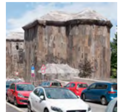
Ibrahim Mahama Check Point Sekondi Loco
